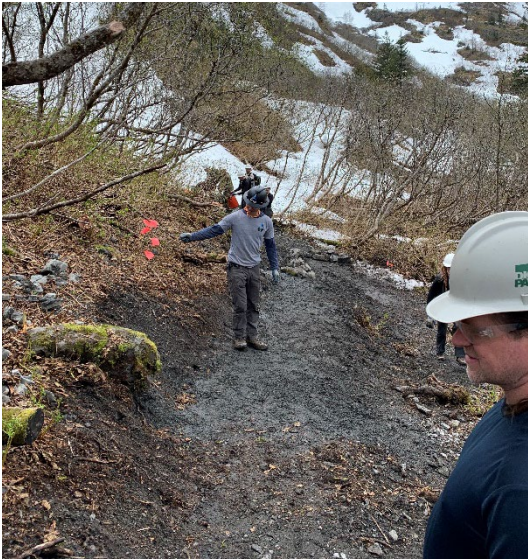
Before and after shot on the Horsetail Falls Connector Trail. Trail was rerouted to have a more sustainable grade.
