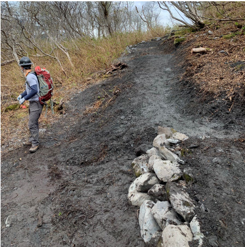
View from bottom of trail reroute. Rock wall in lower half of picture was built to get around exposed bed
