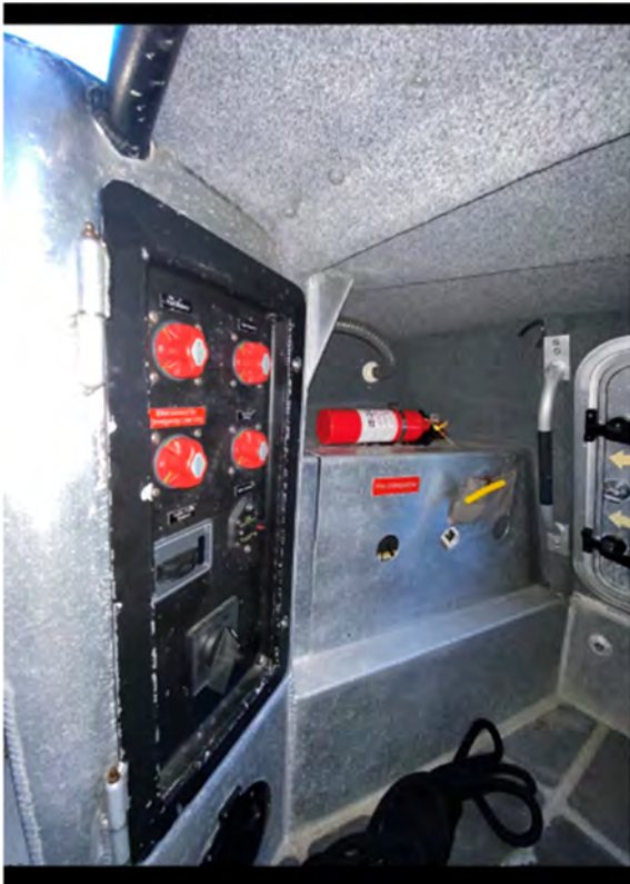
PHOTO OF INTERIOR:
