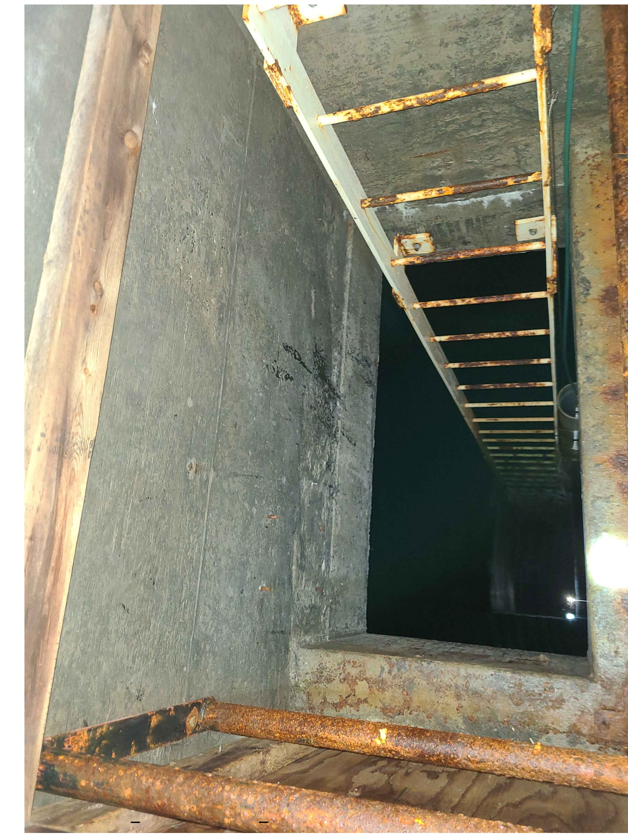
2 EXHIBIT PHOTO OF LOOKING INTO RESERVOIR
