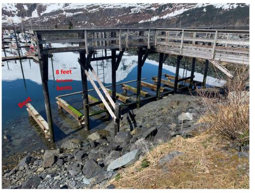
A vessel that has a 5ft draft will need at a minimum of +10.5ft tide to get on and off the grid.
