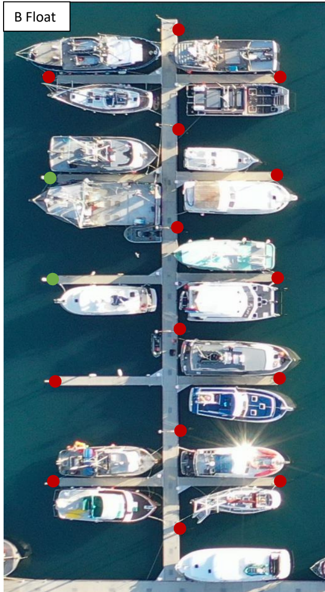
B Float – 14 Wood Piles 2 Steel Piles
